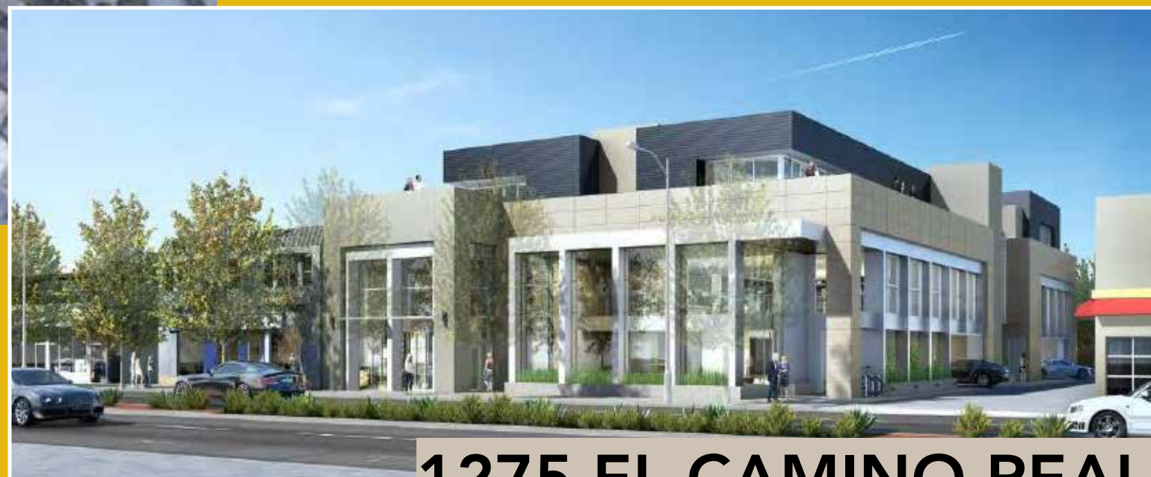
E 1275 EL CAMINO REAL 3 Residential Units / 9,378 SF Office / 612 SF Retail Status: Under Construction
